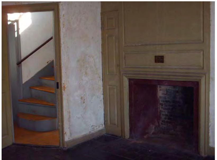
Kitchen Chamber: note plain molding, fireplace surround, and white plaster walls
