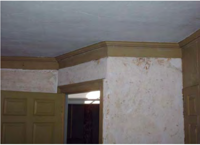
Ceiling molding and plaster walls
